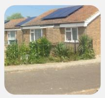
These bungalows (above, far left and left) needed different measures and received cavity wall insulation, loft insulation, air source heat pumps and solar panels to improve their energy efficiency.
