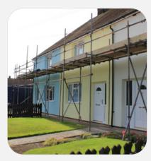
These solid wall homes (above, left and right) received external wall insulation, triple glazed windows, new roofing, loft insulation and solar panels.
